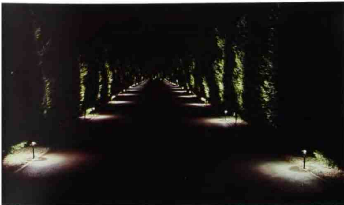
below: Uplighting and spreadlighting at intervals along this 120m (400ft) driveway lined with Cupressus Leylandii conspire to provide ornamental access lighting.
