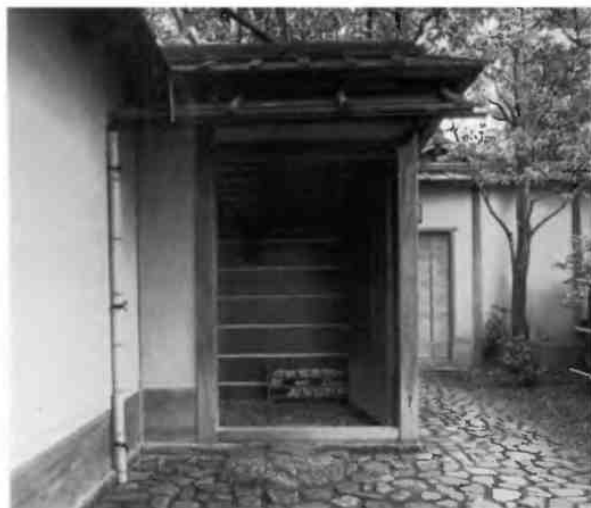
Roji-mon, the narrow, covered entrance gate to the tea garden proper. Its approach is paved with large round cobbles of natural stone.
